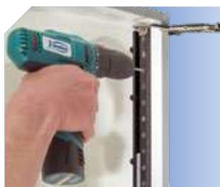
Drilling for placing shelves.
