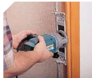
Fitting hinges with the CPN66 head.
