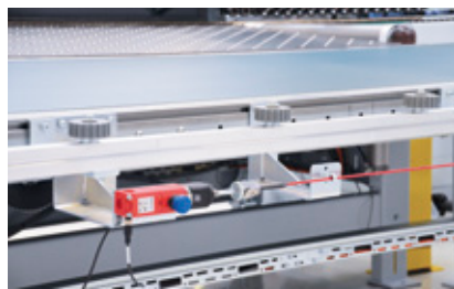
Equipment to achieve CE-conformity: rip cord back to the return belt
